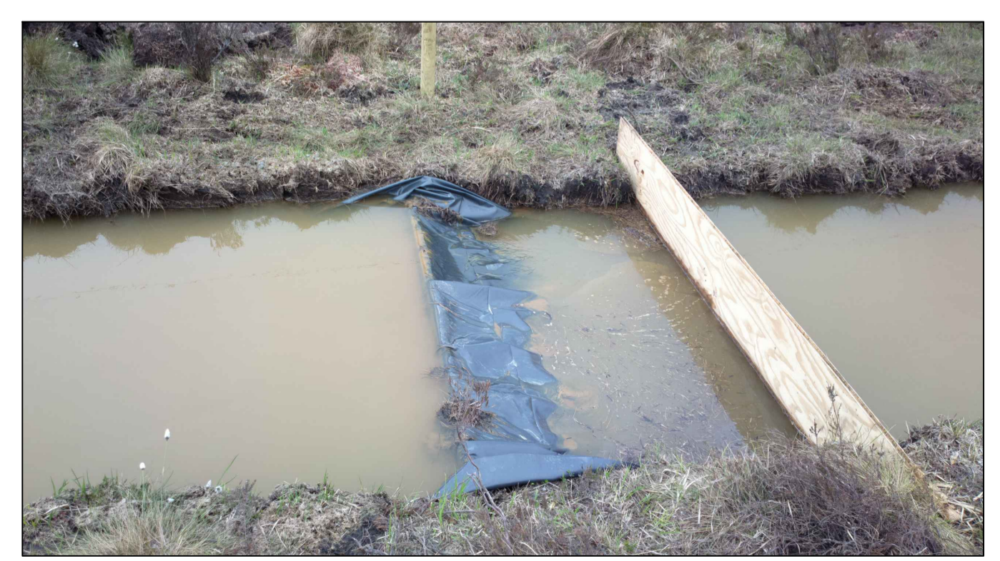
Baffle/Weir Detail
