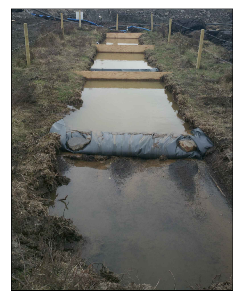
Completed Settling Pond System
